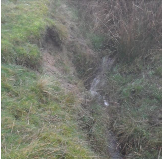
Photo 3.4: Minor waterfall in dredged section between OSB and CSB
