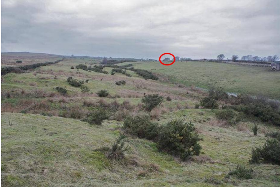
Photo 3.1: Middle section of Matthew Dike (looking upstream)
